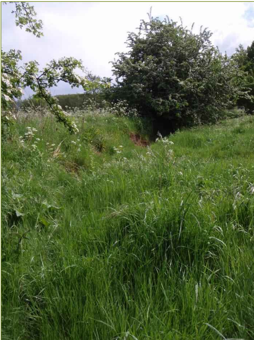
29. Old drainage ditch with scrub growing within it
