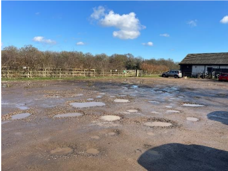
Figure 7 Car park surface
